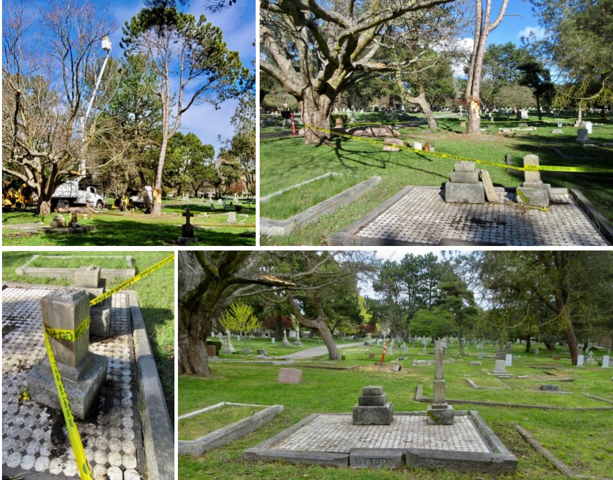
March 25, three views; lower right, April 12, after repairs. Photos by Diana Pedersen and Yvonne Van Ruskenveld
