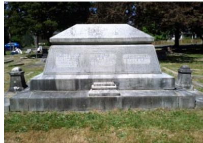
Wilson mausoleum after cleaning
